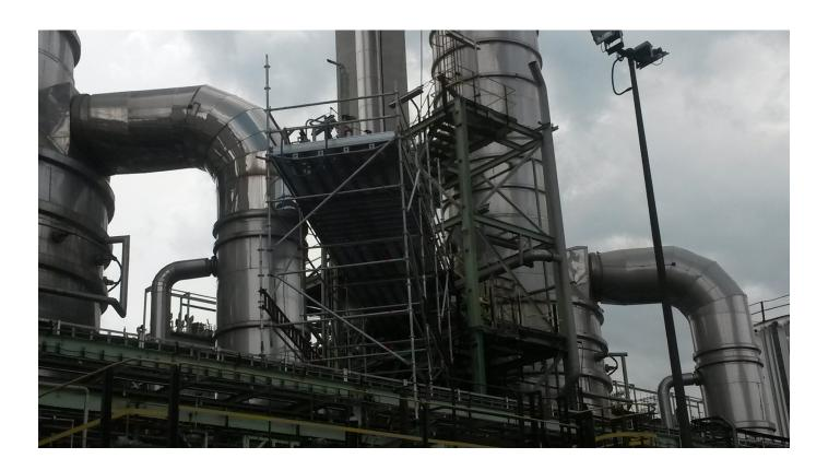
GBM Network also applauded how easy it was to use the Layher Scaffolding System. Diagonal braces ensured a straight scaffold with no couplers on braces and their boards also carried less sand from sand blasting.
